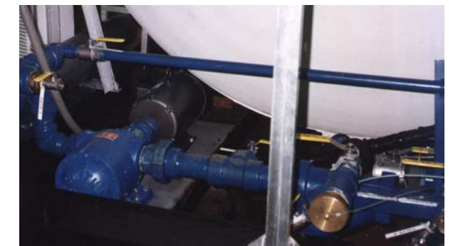
Built in liquid CO2 transfer pump (left) and main outlet connection with valves (right).
